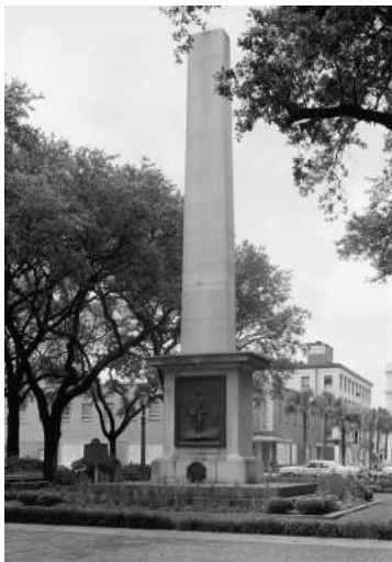
Greene Monument and Grave, Savannah (Historic American Buildings Survey via Wikipedia)
